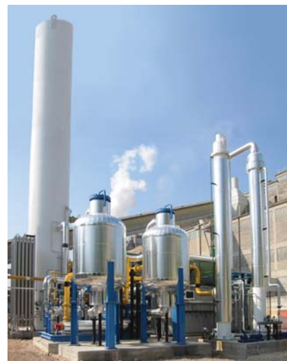
Impianto OxyCEMENT 1500 - Italy
